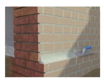
b) Existing, Adequately Load-Bearing Bituminous Waterproofing Clean the existing bituminous waterproofing layer, ensuring it is well-adhered to the substrate and structurally sound. Apply a bonding layer by scratch-coating the surface with **BOLIX H-HYBRID** compound, extending at least 20 cm beyond the designated fillet area.
