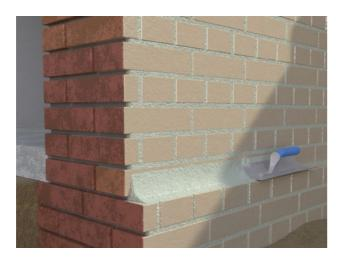
b) Existing, sufficiently load-bearing bituminous waterproofing Clean the existing bituminous waterproofing layer, ensuring it is well-adhered and structurally sound.
