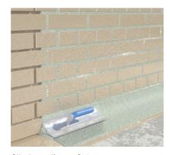
on-wet method. Maintain a minimum fillet radius of 4 cm.
